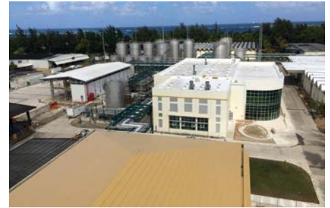
Bacardi Spirit Manufacturing Facility Catano, Puerto Rico
