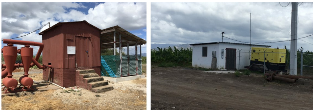
Figure 3-11: Water Wells at Agricultural Biotechnology Farm Operations in Juana Diaz, February 2018. Left, Permanently Installed Backup Generation; Right, Temporary Generator Operating Well at an Agricultural Biotechnology Farm Operation (Photos by Matthew Berry/Argonne)
